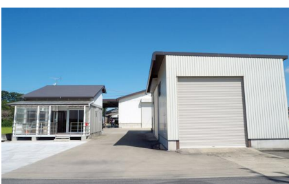
Appearance of the Factory
